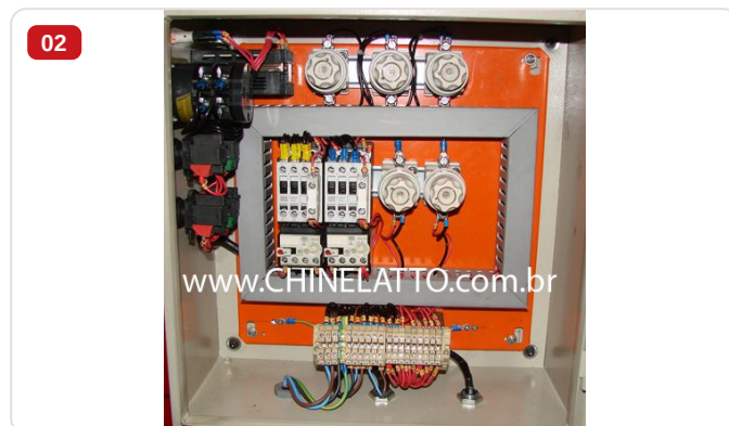
Detail — Electrical panel of BB-98 honing machine with contactors and relays for industrial automation
